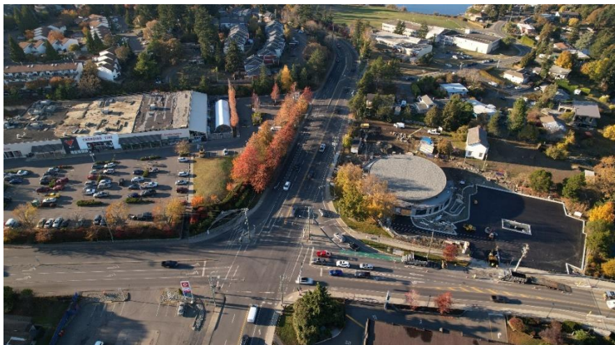
The three critical corridor improvements: Admirals Road (top left), Helmcken Interchange (top right), and Island Highway (bottom)
