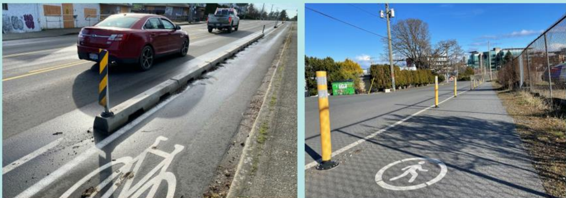
Examples of quick-build facilities with protected bike facilities on Tillicum Road in Saanich (left) and an adaptive sidewalk on Langford Street in Victoria West (right).
