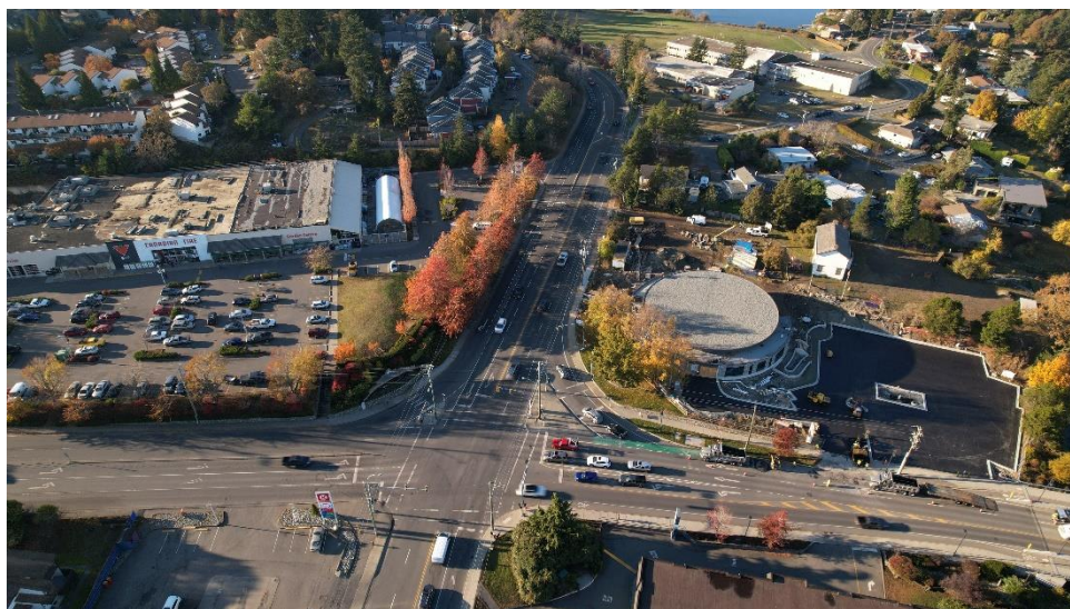
The three critical corridor improvements: Admirals Road (top left), Helmcken Interchange (top right), and Island Highway (bottom)
